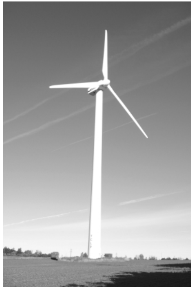
Wind turbine, Traverse City Light & Power
